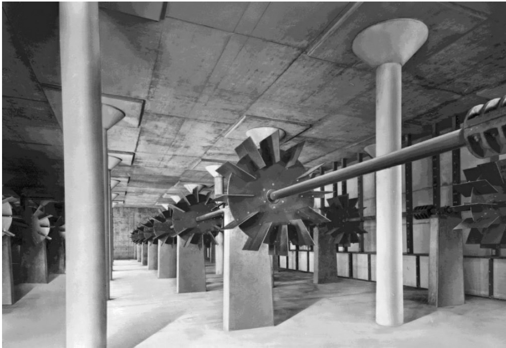
FIGURE 6.18 Turbine-type flocculators. ( Courtesy of Envirex, a Rexnord Company. )
